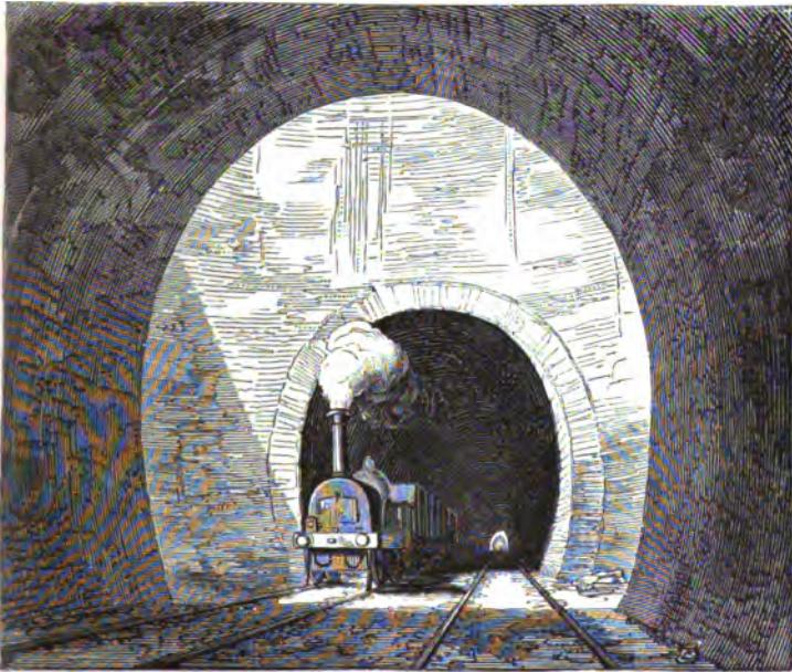
SHAFT OF KILSBY TUNNEL.
